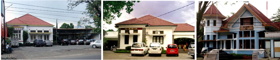
Picture 6: Some old buildings which already changed to be commercial buildings.
