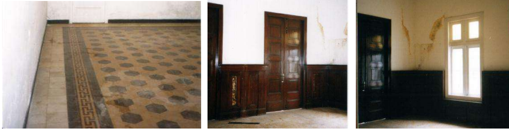
Picture 8: Details of floor tile and interior existing.
