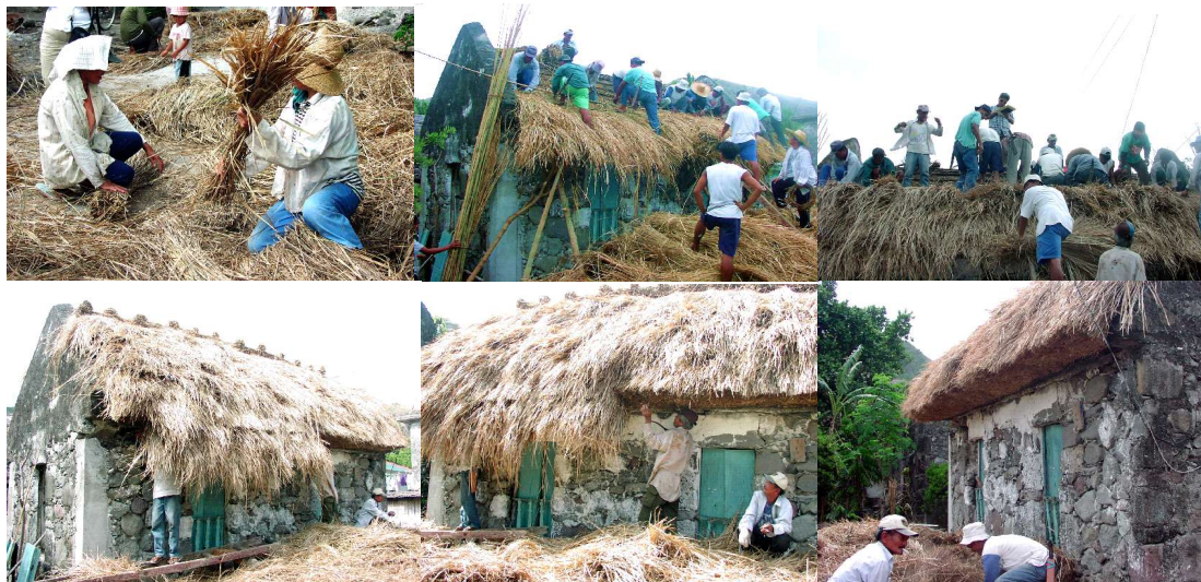
Fig. 19 to 24 – Kama idungan Cooperative’s Re-Roofing Activity
